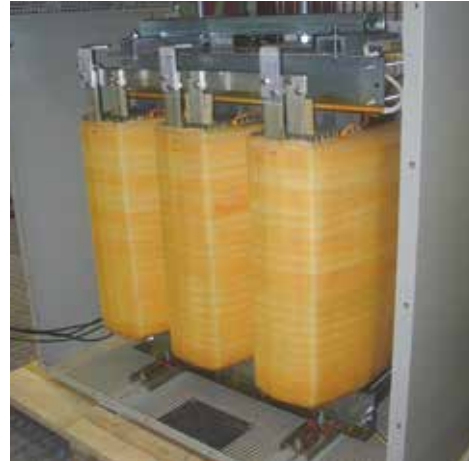
400kVA with aluminium windings
